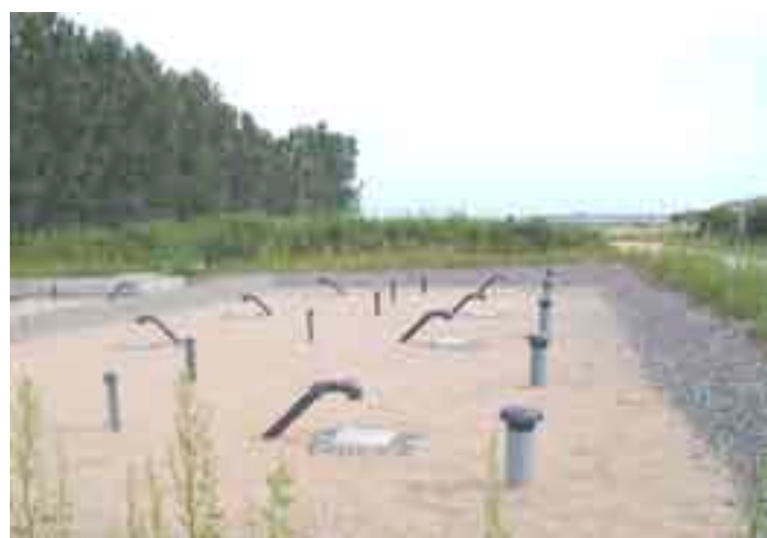
Figure 6: First stage bed just after completion and before reed planting (Photo: Liénard, 2003)
